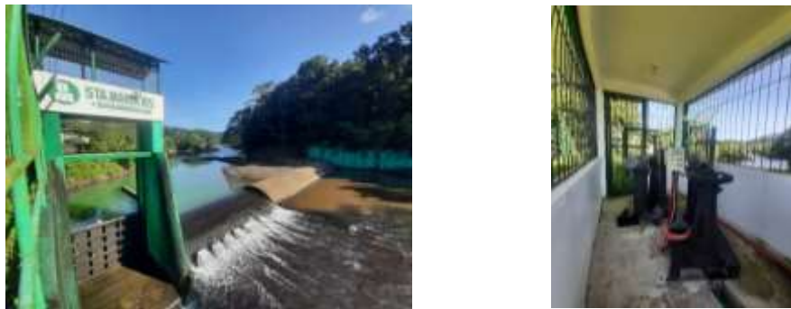
Figure 1. Bagumbayan Dam intake gates of Sta. Maria RIS
